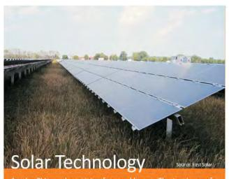
A solar PV panel consists of several layers. The top layer of glass provides weather protection for the PV cell. A special coating is applied to the glass to reduce reflected light from the panel, thereby reducing glare. Within the solar PV cell is a grid, often made of metal which conducts electricity.
