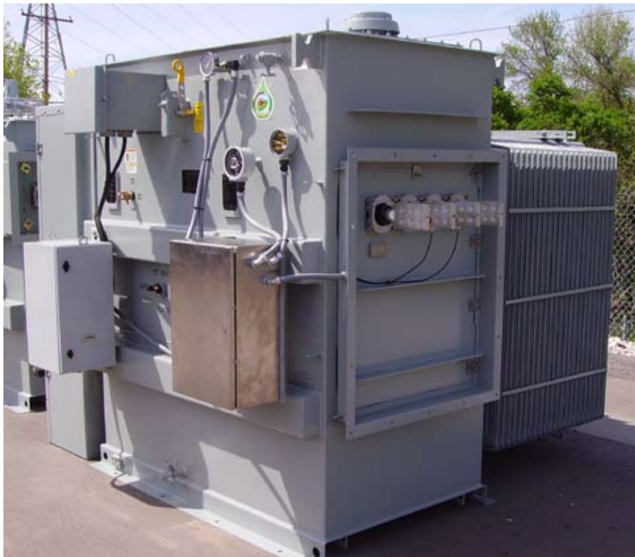
Figure 1. Unit type substation transformer equipped with low-voltage transition flange and high-voltage full height air terminal chamber.
